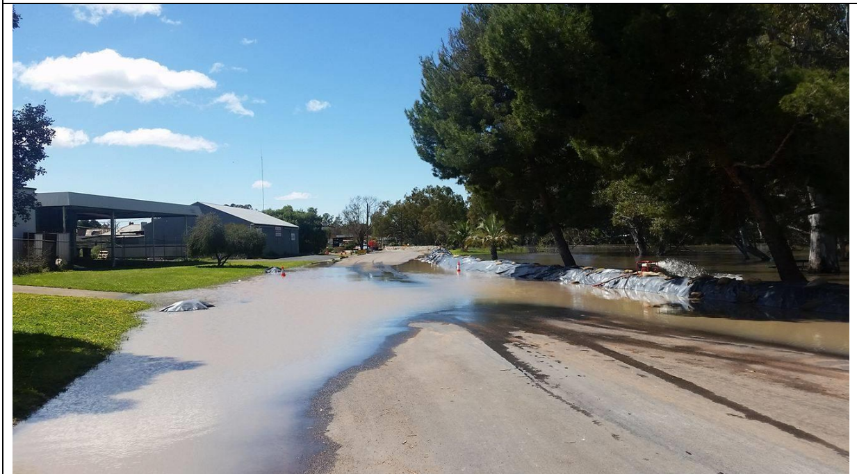
Plate 2 – Looking east at section of temporary levee at corner of Lachlan and Denison Streets
