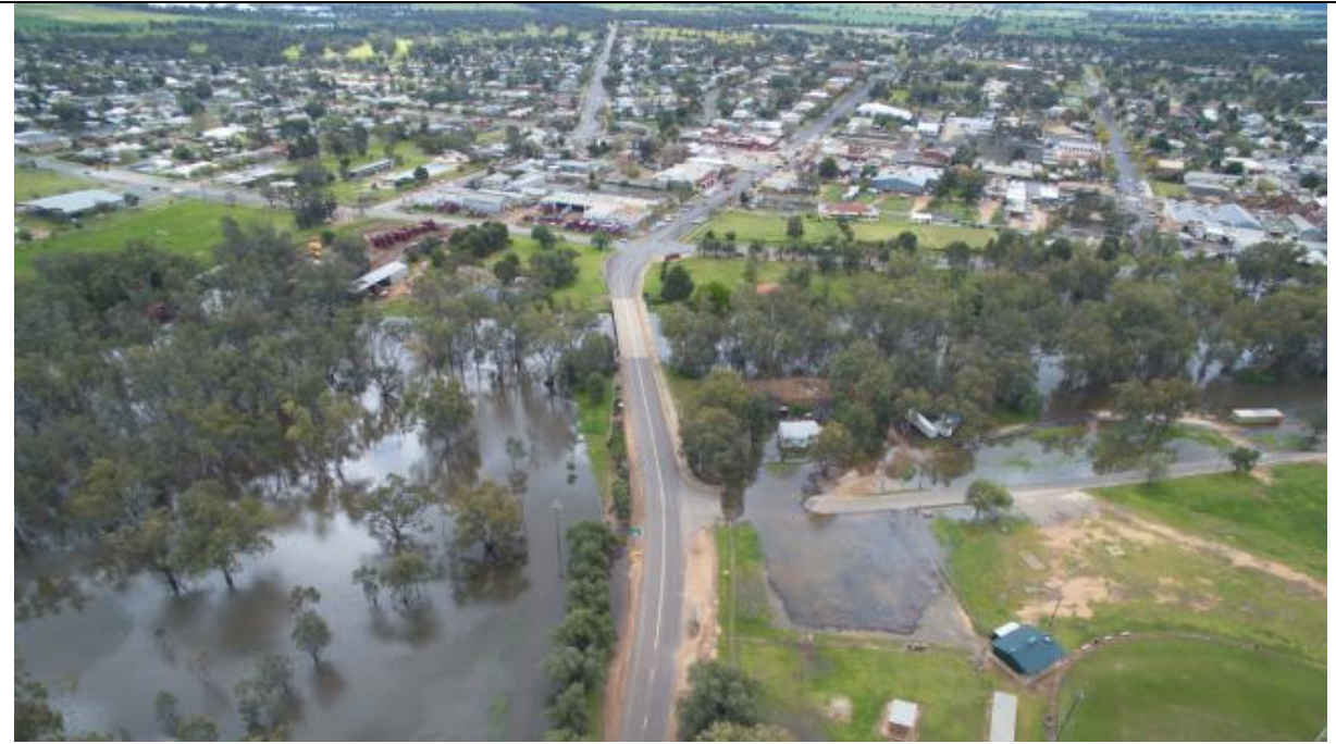
Plate 7 – Looking North along Diggers Avenue at Condobolin Bridge
